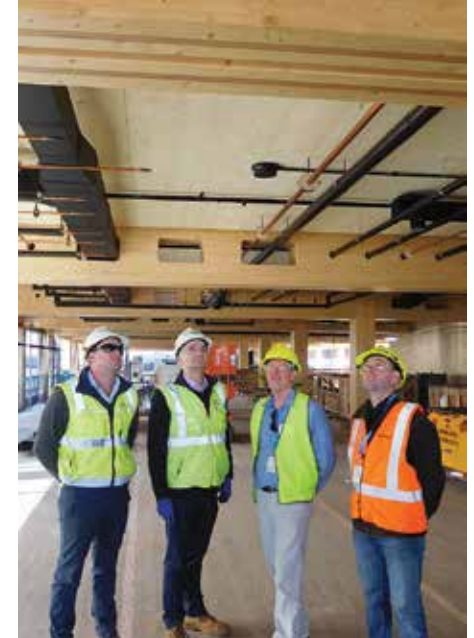
Lendlease construction manager David Elliott and site manager Oliver Close point out CLT components at International House in Sydney to AFS site tour members David West, general manager, stewardship, HQPlantations, and Tim Cleary, skills advisory manager, ForestWorks.
